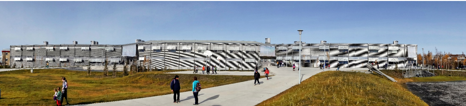
Exterior Ramp, East Three Schools, Inuvik
